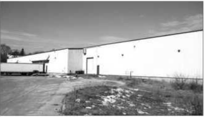
INDUSTRIAL-SUB-LEASE: Woonsocket, 30,750' High Bay Distribution Warehouse, with 4 tailboard docks, 20'-27' clear height.
