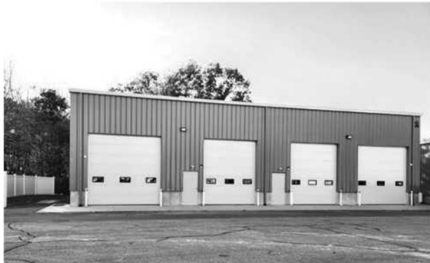
Seths Way/39 Nooseneck Hill Rd (Rt 3) West Greenwich, RI - just 1/2 mile from Rt 95, planned business park coming soon with units from 4800-24000 sq ft. will finish to suit from $12. psf/yr plus
