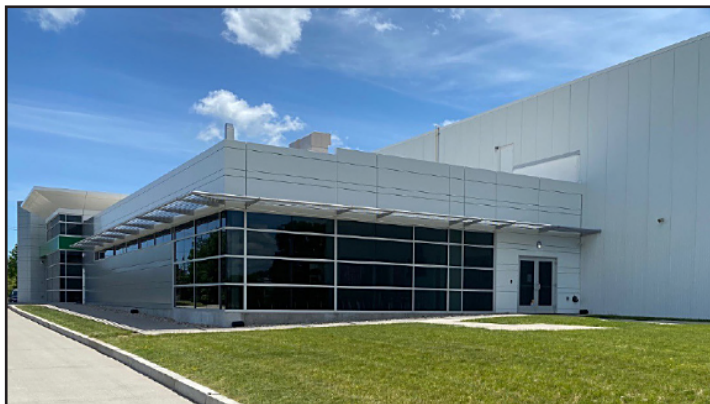
81 Ocean State Drive, Quonset Business Park - North Kingstown, RI
