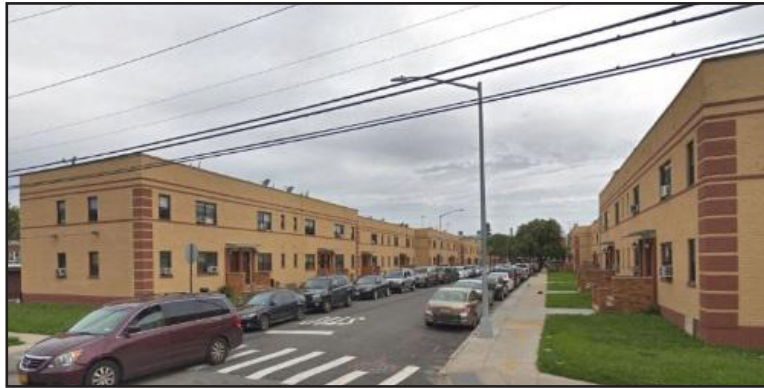
102-04, 102-34 and 102-31 184 th Street - Queens, NY
