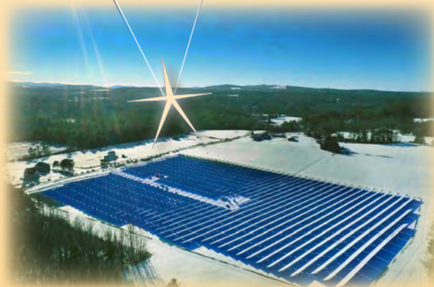
7MW Solar Field, China, ME
