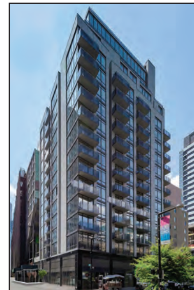
42-10 27th Street - Queens, NY
