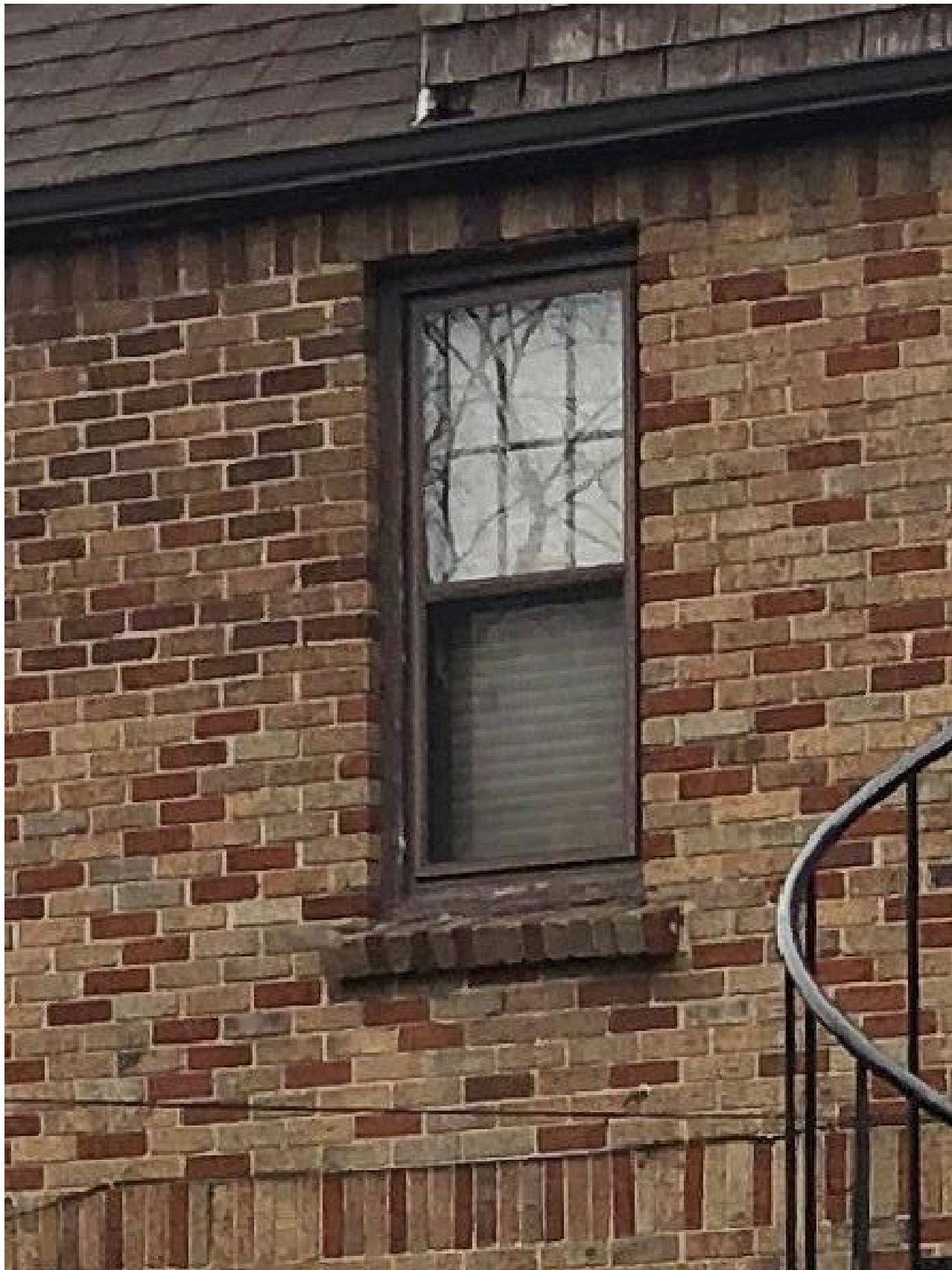
EXISTING BRICK WINDOW SILL DETAIL REFERENCE
