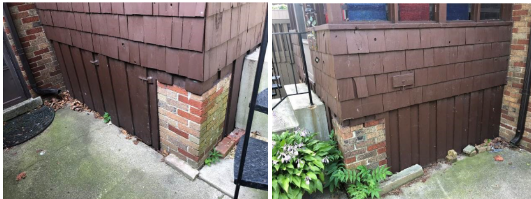
Similar brick used on both exterior facade of main building and pilings for the rear enclosed porch.
