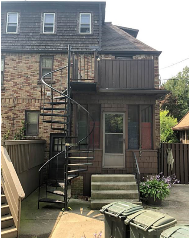
View of rear attached enclosed porch and fire escape staircase which is to be removed.
