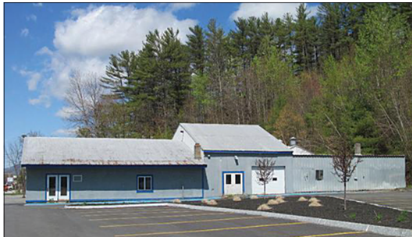
PRIME VISIBILITY, (20k cars per day), across from Market Basket, Hobby Lobby, State Liquor Store & TJ Maxx. 6300 square foot bldg w/5 overhead doors, offices & service areas plus detached 936 square feet w/3 bays. $419,000
