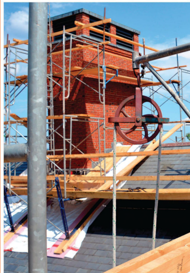
Historic Roof Restoration | Cambridge, MA
