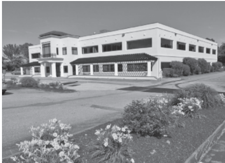
Swansea $Upon Request Recently renovated, flexible size of space available for lease, 4000 sf to 16,500 sf. Ben Edgar 508.776.2635
