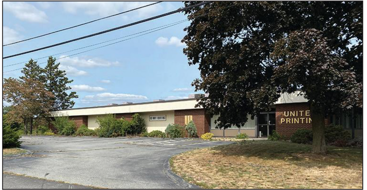
55 Colorado Avenue - Warwick, RI
