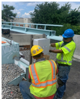
Crew installing stray current on GLX
