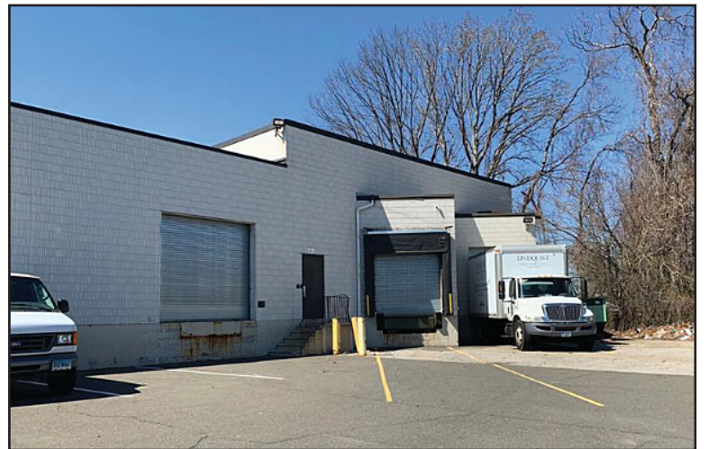
240 Hathaway Drive - Stratford, CT
