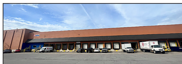
The Concourse Center at 4039 Genesee Street - Buffalo, NY
