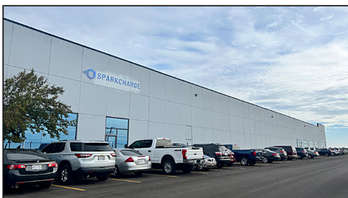
The Concourse Center at 4039 Genesee Street - Buffalo, NY
