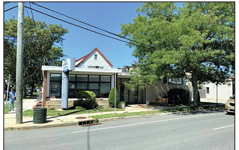
192 Hillside Avenue - Williston Park, NY
