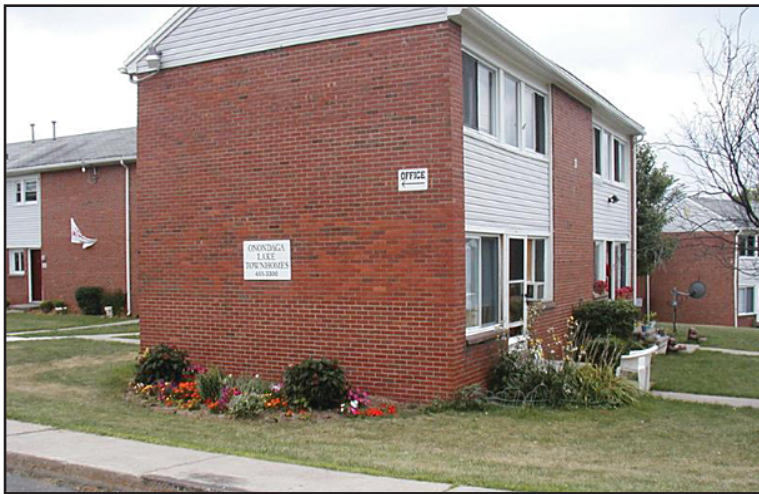
Onondaga Lake Townhomes, 151-159 Old Liverpool Road - Liverpool, NY
