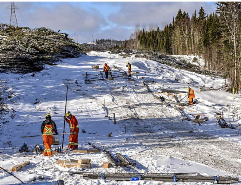
..... Assembly crew laying out tower steel (left) and assembling body of guyed structure (right). Credit: Valard Construction.
