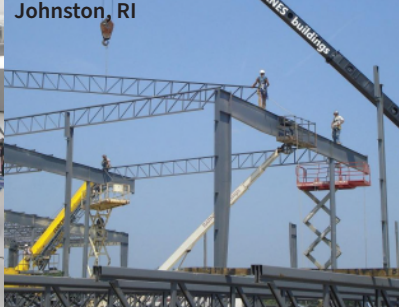
Fed Ex Distribution Center Johnston, RI
