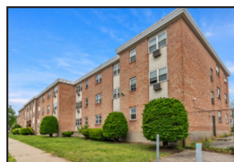
Westnor Apartments, 45 Monroe Street - Bridgeport, CT
