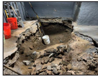
Start of remediation of floor.
