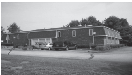
Brick Office Building for Sale
