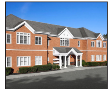
325 Meeting House Lane - Southampton, NY
