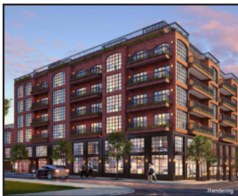
25-16 37 th Avenue - Long Island City, NY
