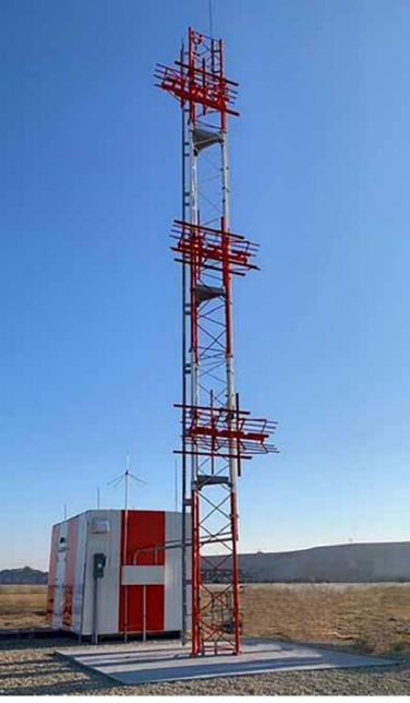
Instrument Landing System (ILS) installed at Marshall Army Airfield, Fort Riley, KS.
