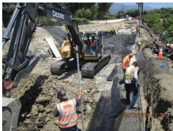
Workers install lightweight TDA fill to prevent the ground under the road from slipping.
