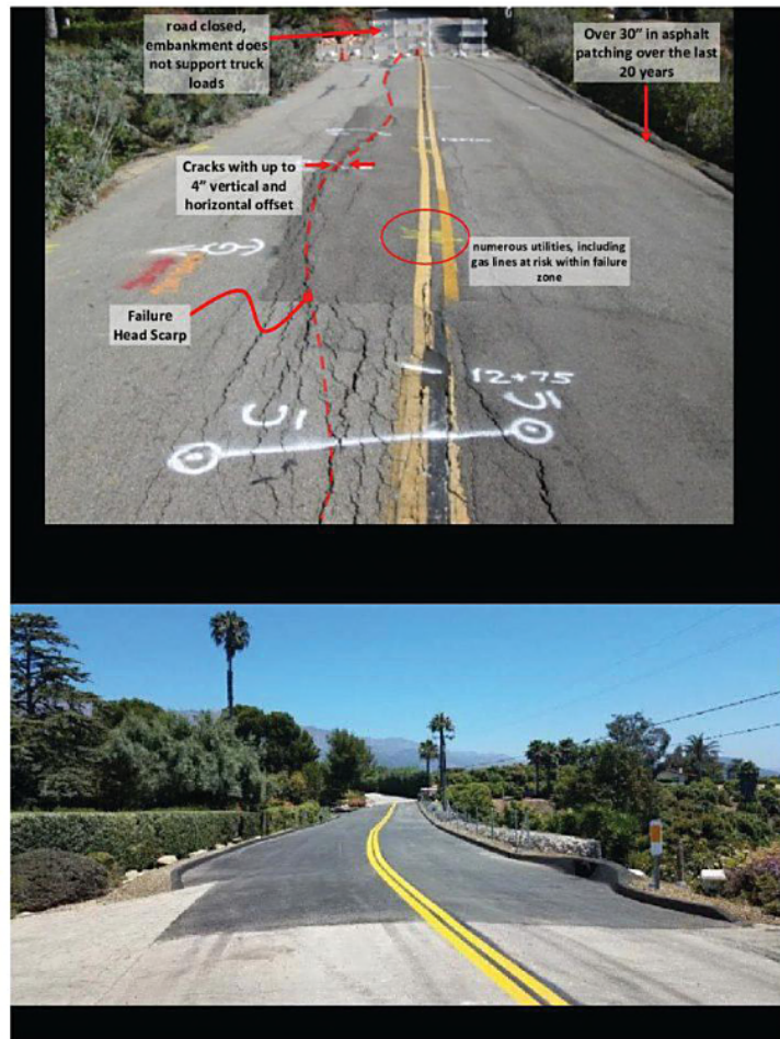
Engineers identified road conditions prior to repair (top). Completed road (bottom) after embankment reconstruction using TDA.
