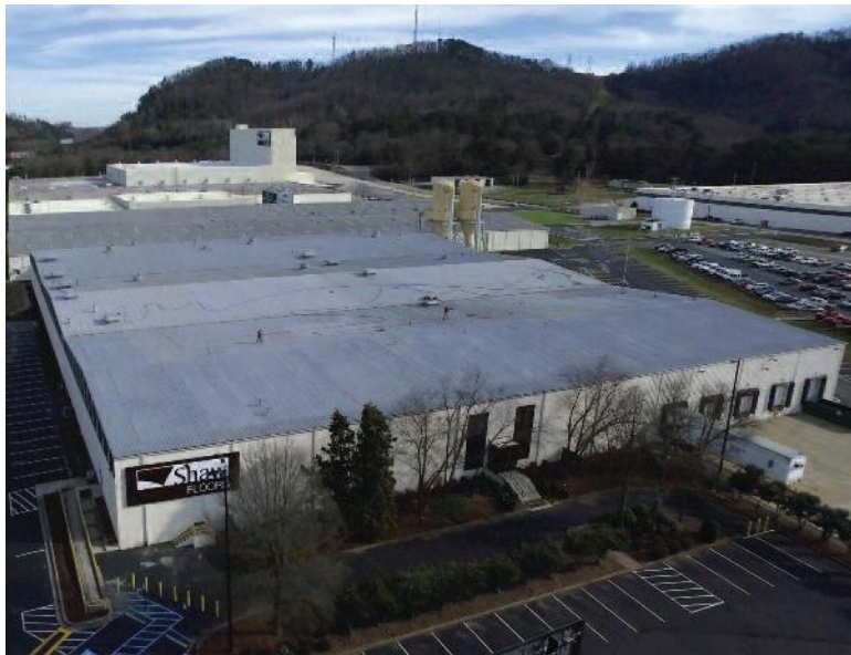
Shaw Floors' Plant RP in Ringgold, Ga., has the capability to produce rigid core products.
