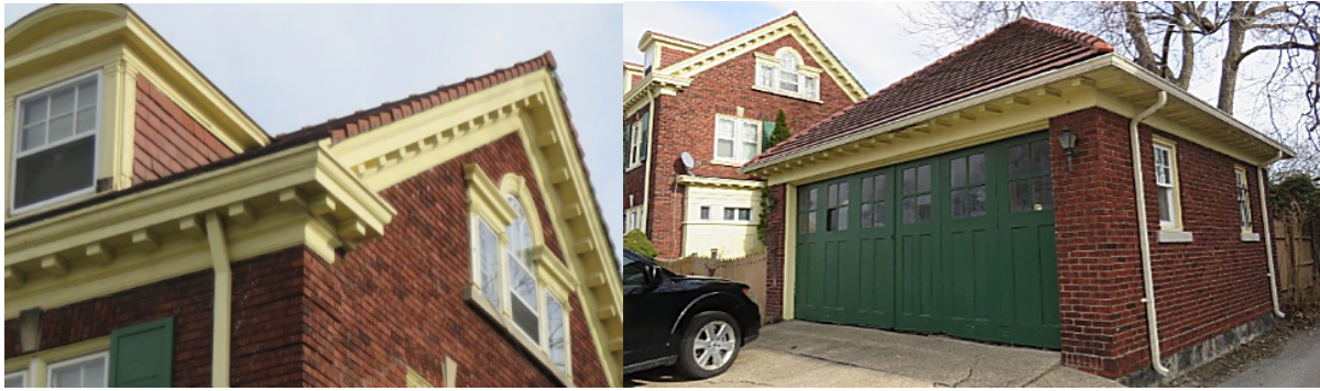
Compare appearance of original existing integral eavestrough on main building (on left) versus new types of eavestrough system on garage building (right)
