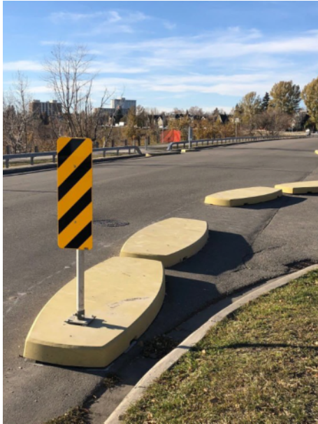
Figure 1: Temporary Traffic Calming Curbs (source: City of Calgary)
