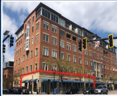
Walgreens Retail Condo Boston's Historic South End | $6,810,000
