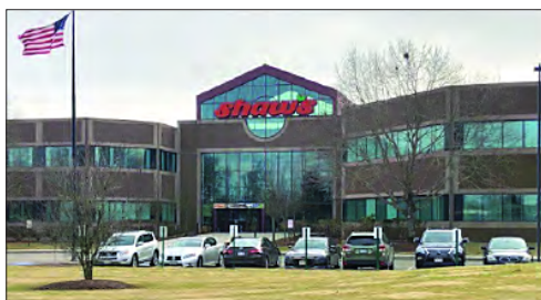
FOR LEASE - W. BRIDGEWATER 19,000 SF Plug & Play Office Space Full building generator - cafeteria .3 Miles to Route 24
