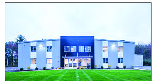
FOR LEASE - W. BRIDGEWATER 16,000 SF± 17' Ceiling Height 2 Docks - 1 Drive In
