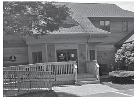
Mashpee $149,000 2,919 sf office condo in Shellback Place on Barnstable/Mashpee town line. 2nd floor unit. John Callahan 508.737.1322
