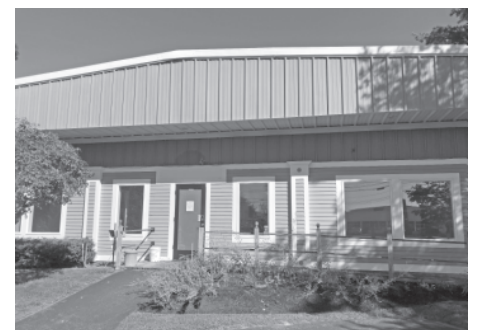
Falmouth $14/sf/yr/ NNN Unit A -5 offices, conference room & storage. Unit B -1 office, studio & storage. Fox Team 617.529.8616
