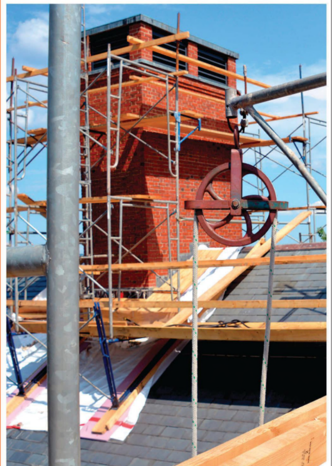
Historic Roof Restoration | Cambridge, MA
