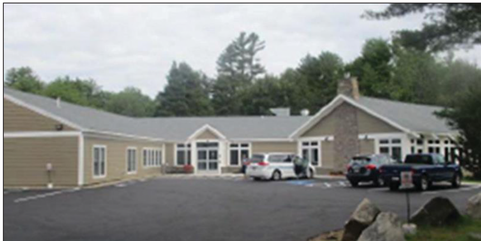
51 Main Street - The Lodges Care Center - Springvale, ME
