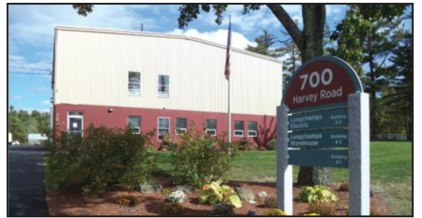
700 Harvey Road - Manchester, NH
